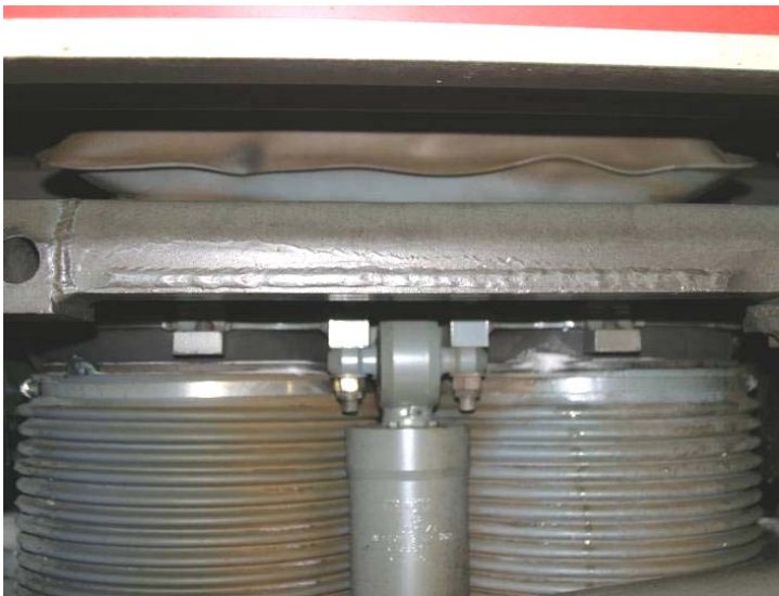
Figure 13. Snow covers both for the secondary coil springs and for closing the gap between the car body and the bogie frame at the Finnish Sm3.
