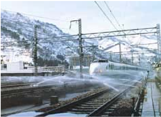
Figure 30. A Japanese water sprinkler system in practice 15 .
