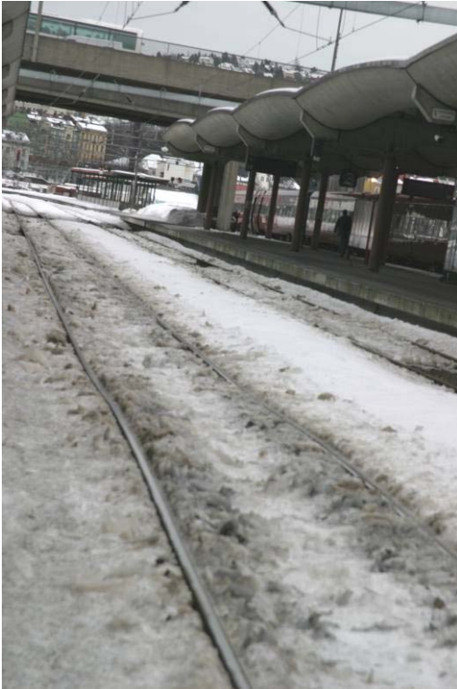
Figure 35. A platform track with a lot of ice that has fallen of stopping trains.
